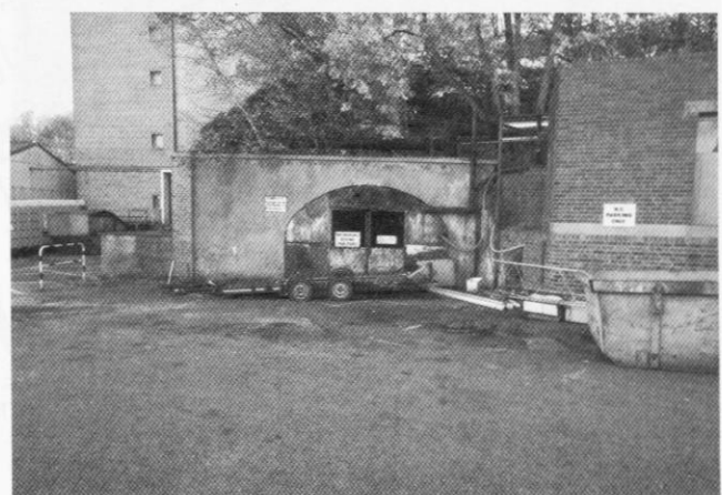
Tunnel MT8. Photo by Nick Catford.
